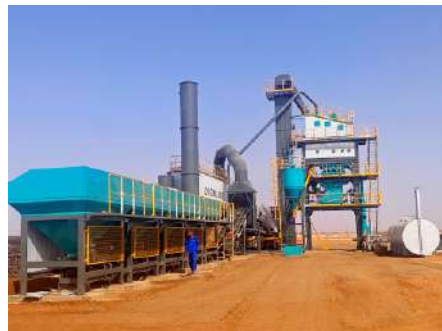
ZAP-S160 Asphalt Plant in Sudan
